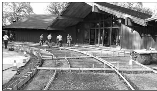
Concrete forms for new entrance, done by A-Z Paving
